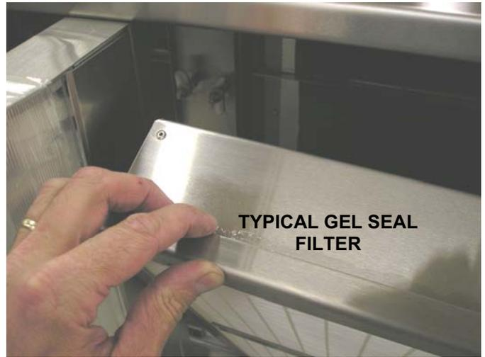
**STEP #2** - POSITION FILTER INTO OPENING OF UNIT
